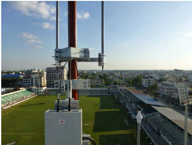
●Photo 1 LTE base station (Soccer stadium in Mandalay)
