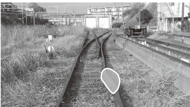
(b) Deformed rail
