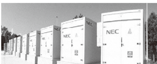
Photo View of the grid storage system.
