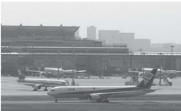
Photo 1 A view of the International Flights Passenger Terminal taken from the domestic flights passenger terminal.
