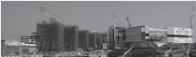
Photo 5 Construction site of the airport terminal building.
