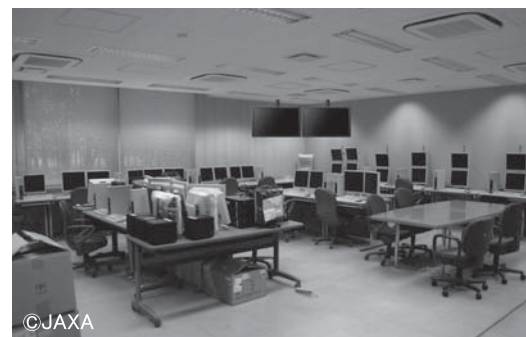
Photo 3 Satellite control equipment.
