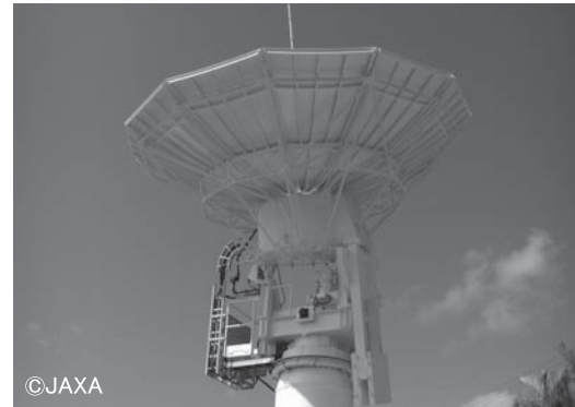
Photo 1 \phi 7.6-meter transmission/reception antenna.
