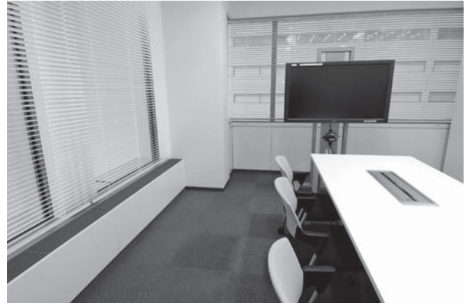
Photo 3 Natural ventilation system, automatic electric shutter blinds and Low-e window glass.
