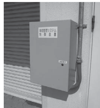
Photo 2 Vehicle management system control unit (image of installation).
