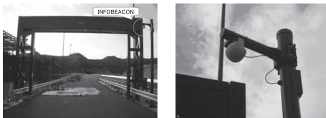
Photo 4 The INFOBEACON installed at the Kakegawa test road site.
