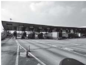
Lok Ma Chau Gate, which is one of the four boundary gates introducing the system.
