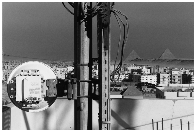
Photo 2 PASOLINK installation site.
