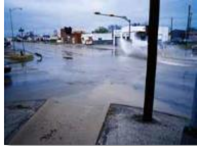
2. Damage caused by flooding in urban areas
