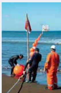
Laying of large capacity submarine optical cable
