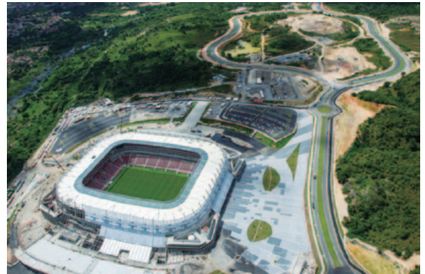
Itaipava Arena Pernambuco under construction
