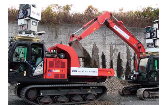
Remote control of construction machinery using 5G
