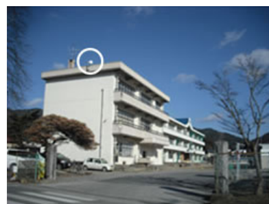
An elementary school building after the installation of network equipment
