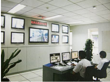
The wireless system control room of the Huichen Senior Service Group
