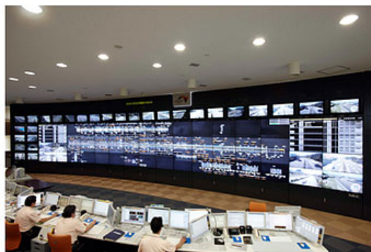
The giant screen at the control center
