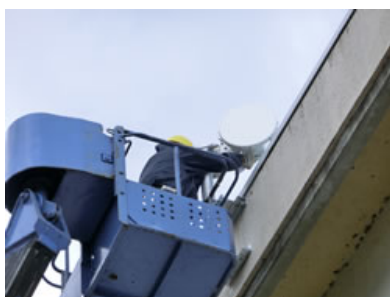
Network equipment is installed on an elementary school building
