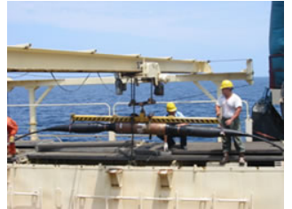
Installation of submarine cable
