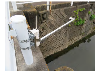
A sensor installed near a riverbank
