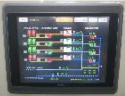
Air conditioning equipment control panel
