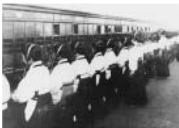
The first large-size common-battery switchboard for long-distance calls was installed in a telephone office opened in Tokyo in 1919 for exclusively handling long-distance calls.
