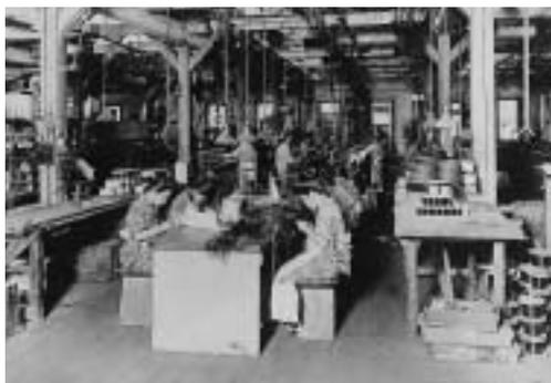
Large volumes of cable were used for switchboards. Most cable production processes were manual. The photo shows a factory scene in the Mita Plant in 1922.
