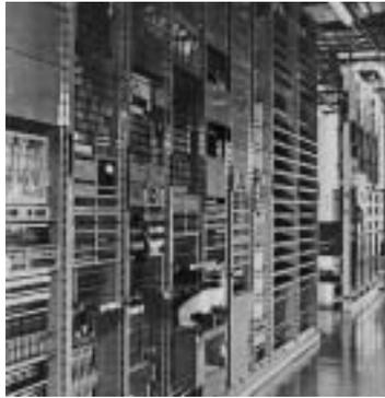
Nippon Electric played a leading role in developing and mass-producing cross-bar (XB) switching systems. Shown here is a model C80 system installed in the Sendai Toll Telephone Office in 1959.
