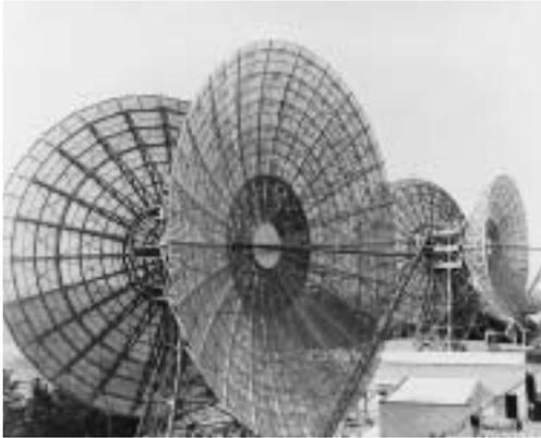
Nippon Electric's over-the-horizon microwave communications technology was highly evaluated at home and abroad. In 1961 the company received a large order from the U.S. Air Force to construct a network connecting military facilities in Japan, Okinawa, and South Korea. The repeater station at Oura in Kagoshima Prefecture connected Okinawa with mainland Japan.
