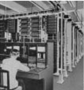
Nippon Electric exported its first domestically produced H-type automatic switching system to Manchuria in 1936. The second H-type system, shown here, was installed in the Hirano Telephone Office in Osaka in 1938.
