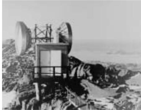
The photo shows an unmanned communications repeater station in Greenland. Great difficulties were met in maintaining and operating such stations in sub-zero temperatures. Nippon Electric developed low-power consumption equipment that required less fuel supply.
