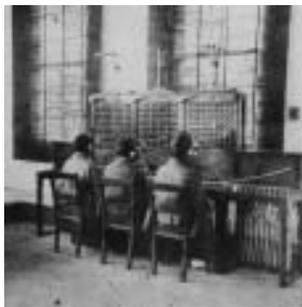
Three telephone switchboards, manufactured in Japan based on the standard switching system of Western Electric (WE), were installed in the Tokyo Telephone Office in 1890 to serve 155 telephone customers.
