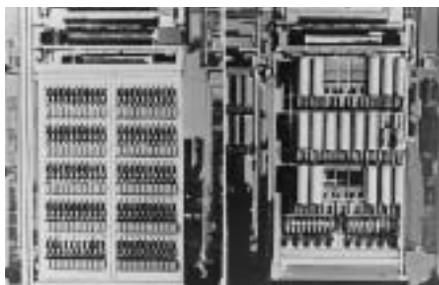
Nippon Electric produced Japan's first domestic-made A-type automatic switching system in July 1929 and delivered it to the Nakano Telephone Office in Tokyo. Service began using the switching system in March 1930.
