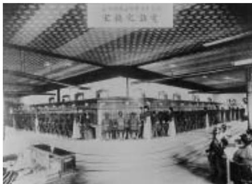
Telephone operators work with parallel duplex switching systems at the Naniwa Branch Telephone Office in Tokyo.
