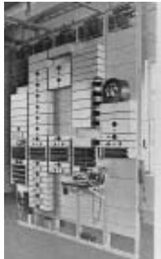
Nippon Electric developed a nonloaded cable carrier transmission system entirely with domestic technology and installed it in 1937 in Manchuria. Shown here is the terminal equipment in the Mukden Telephone Office.
