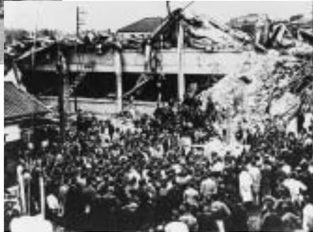
The Great Kanto Earthquake struck the Tokyo-Yokohama area in September 1923. Even earthquake resistant buildings in Nippon Electric's plant were destroyed. The second and third stories of 3-story reinforced steel buildings collapsed (top). Workers in silent prayer after initial rescue efforts (right).
