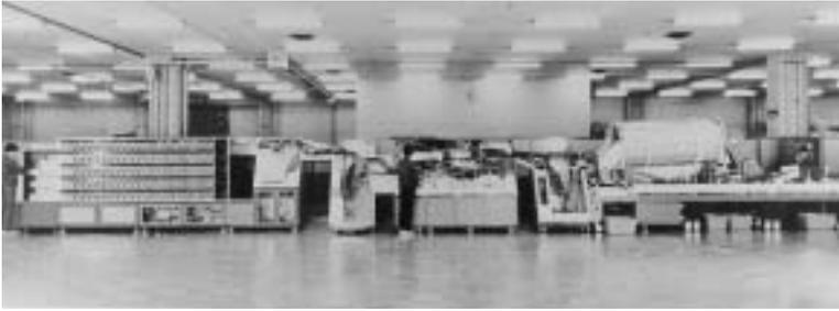
The photo shows the NS-100 fully automated mail processing system undergoing a final test at the Fuchu Plant in 1971. It handled mail in a sequence of cull and face, postage stamp franking, ZIP code reading, and mail sorting functions.
