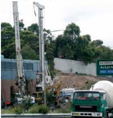
Construction on the Gore Hill Freeway.
