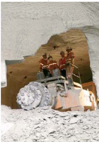
Thiess John Holland workers and a road header machine after the mid-tunnel underground truck loop breakthrough.
