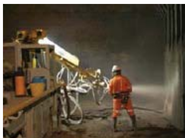
Shotcreting, on the Mowbray Park worksite.
