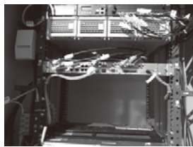
Photo PASOLINK system installation work.
