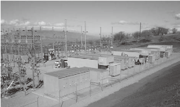
Photo 2 11 MW, 4.4 MWh GSS for stabilizing of wind farm power output in Maui, Hawaii, USA.
