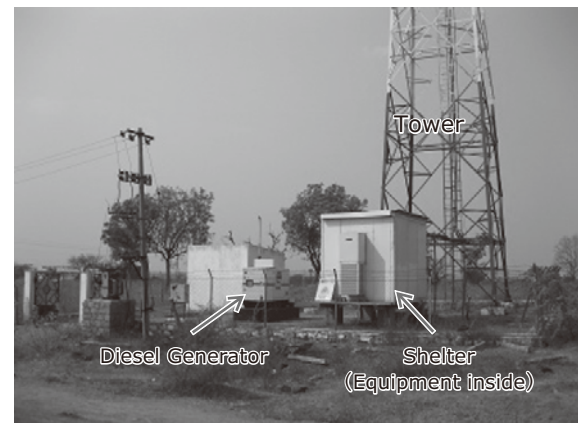
Photo 1 Mobile phone base station (indoor model).
