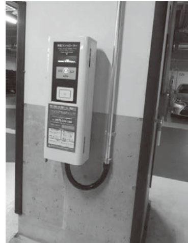
Photo 3 EV charging controller.
