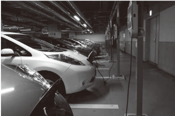
Photo 1 Testing the charging system in Tokyo Midtown.
