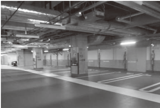
Photo 2 View of the completed charger installation.
