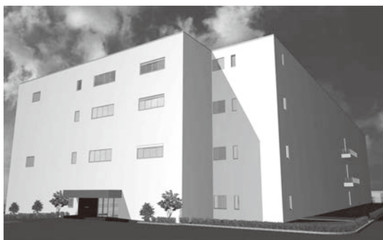
Fig. 1 NEC Kanagawa Data Center.
