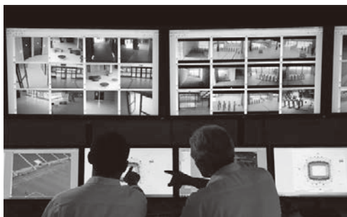
Photo 2 Command Operation Center (CoC).
