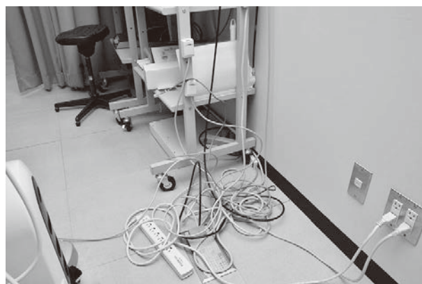
Photo 2 The various LAN ports installed in the medical examination room.
