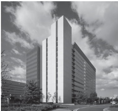
Photo NEC Tamagawa Solutions Center external view.
