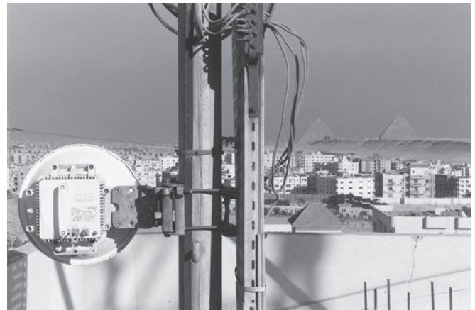
Photo PASOLINK installation.
