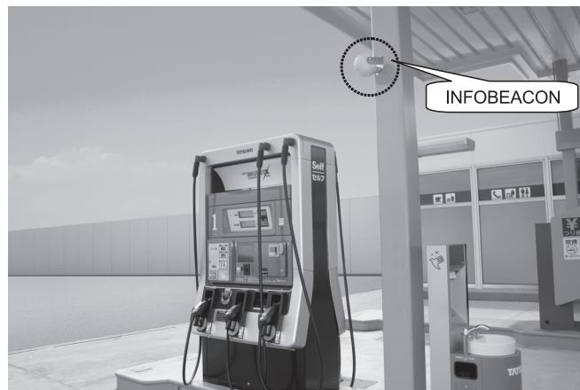
Photo 2 Image of an installation at a gas station.
