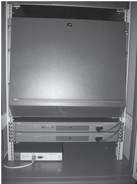
Photo 2 UNIVERGE SV7000 in a 19-inch rack.
