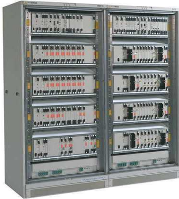
Line Terminal Equipment
