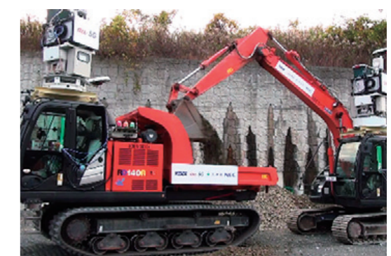
Remote control of construction machinery using 5G
