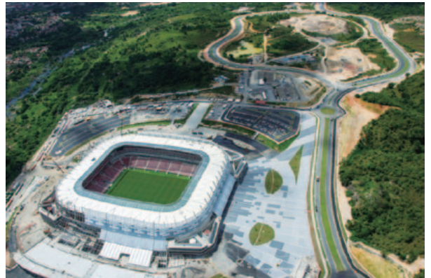
Itaipava Arena Pernambuco under construction
