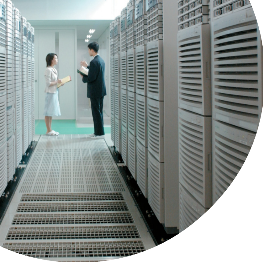
NTT DoCoMo's i-mode gateway system 'CiRCUS.' A prime example of NEC's integrated IT/Network Solutions
