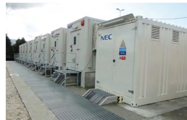
Energy storage system installed in a substation and connected to the actual power grid. The energy storage system covers the balance of supply and demand affected by changes in the solar power and wind power facilities installed in the region.
